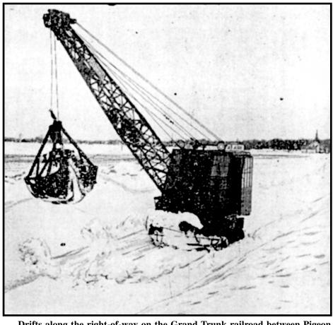
Drifts along the right-of-way on the Grand Trunk railroad between Pigeon (background) and Caseville were so deeply drifted in by snow that workmen were compelled to use a derrick equipped with a clamshell bucket to clear the tracks. A snow plow pushed by three locomotives opened the railroad tracks
